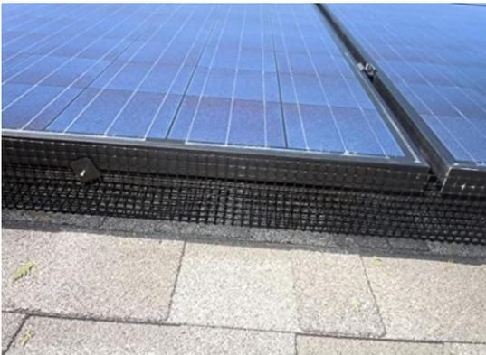
One of the very best ways to control and possibly prevent nesting under your panels is by installing a critter guard mesh. They are anchored along the entire edge of each of your solar arrays. This helps to prevent the birds from getting under the panels and building a nest.
